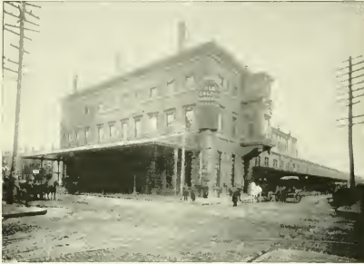
STATION OF OLD COLONY RAILROAD—MAIN DIVISION.
